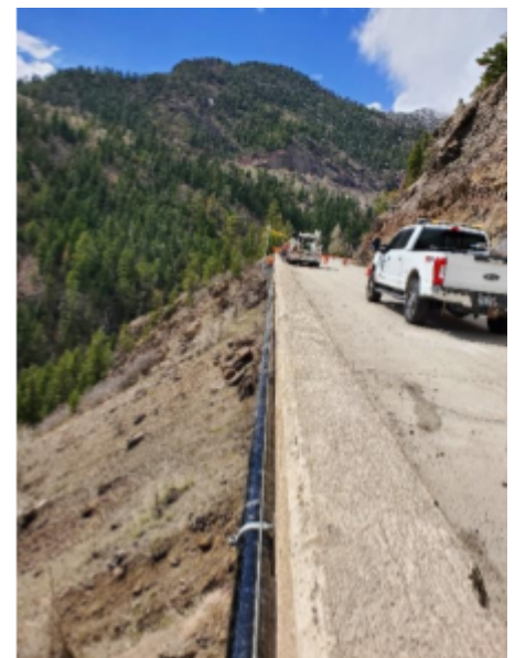
Ongoing trenching activities on US 160 in July 2023.
