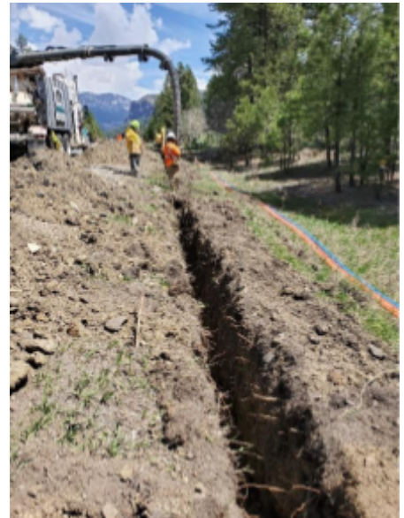
Trenching and directional drilling activities on US 160 in July 2023.
